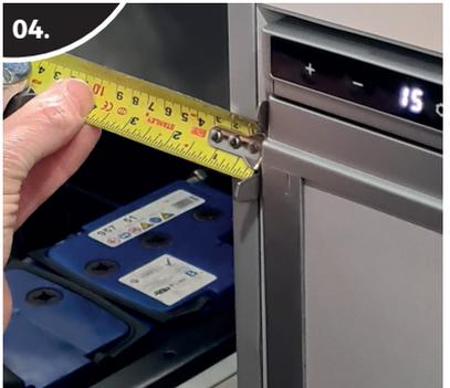
Position the fridge so that it is centred with specified ventilation gaps, be careful to keep the fridge upright and avoid trapping any wires.
